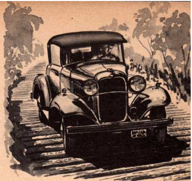
An American car being driven over a corduroy road in the 1930s. In the days before tarmac road surfaces, laying logs across the road in this way was one method of trying to cope with the mud.
